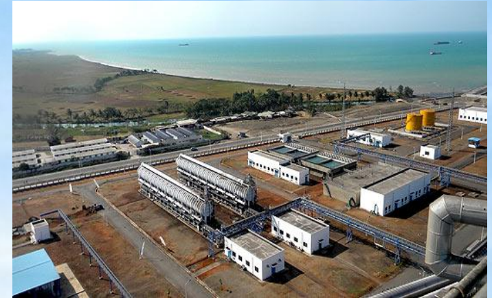
Shanghai Bailonggang Sewage plant (Aisa's largest sewage treatment plant)
