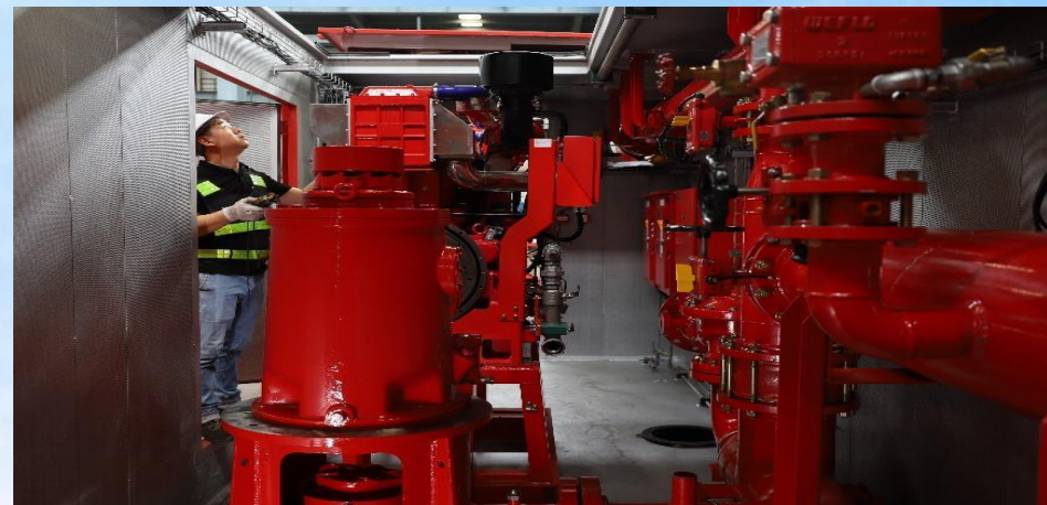
The Sultanate of Oman Khoramabad CCPP & Zan Jan II Power Plant Project
