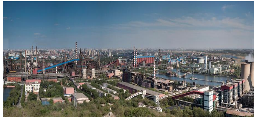
Chongqing Steel Group
